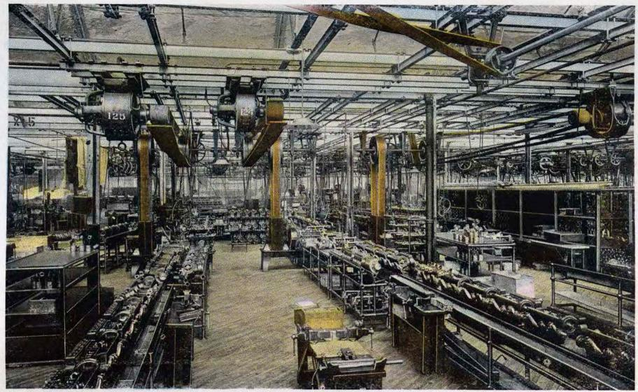
MOVING CONVEYORS HASTEN THE MOTOR ASSEMBLY.
