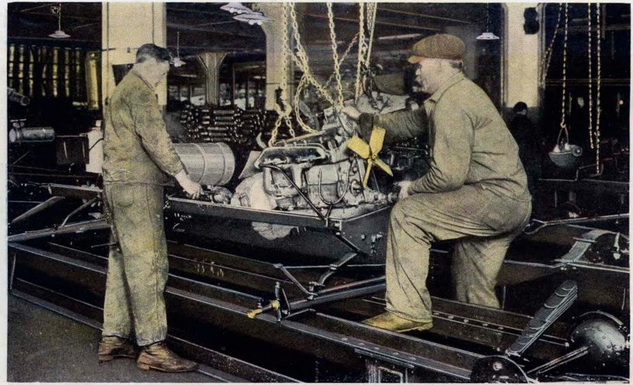
SETTING THE MOTOR, DURING THE FINAL ASSEMBLY.
